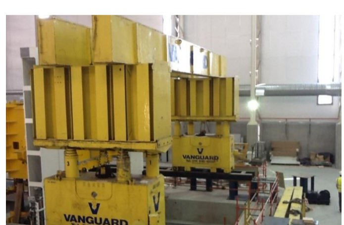
Preparing to lift the crown of the 2 100-ton press which, once assembled, will weigh 297 tons
