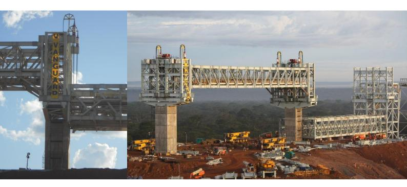
Australian mining company First Quantum needed to assemble two new conveyor sections to columns 60 m above the ground at a site in the Zambian Copper Belt. After months of consultation, it was agreed that instead of assembling the sections at height, they would be assembled at ground level and later lifted by Vanguard to their final positions.
